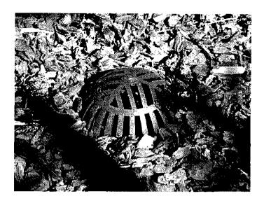
Remove debris from area drains
